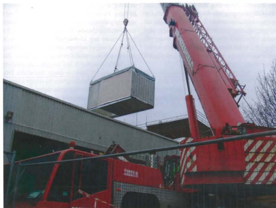
Craning in the modular cell units
