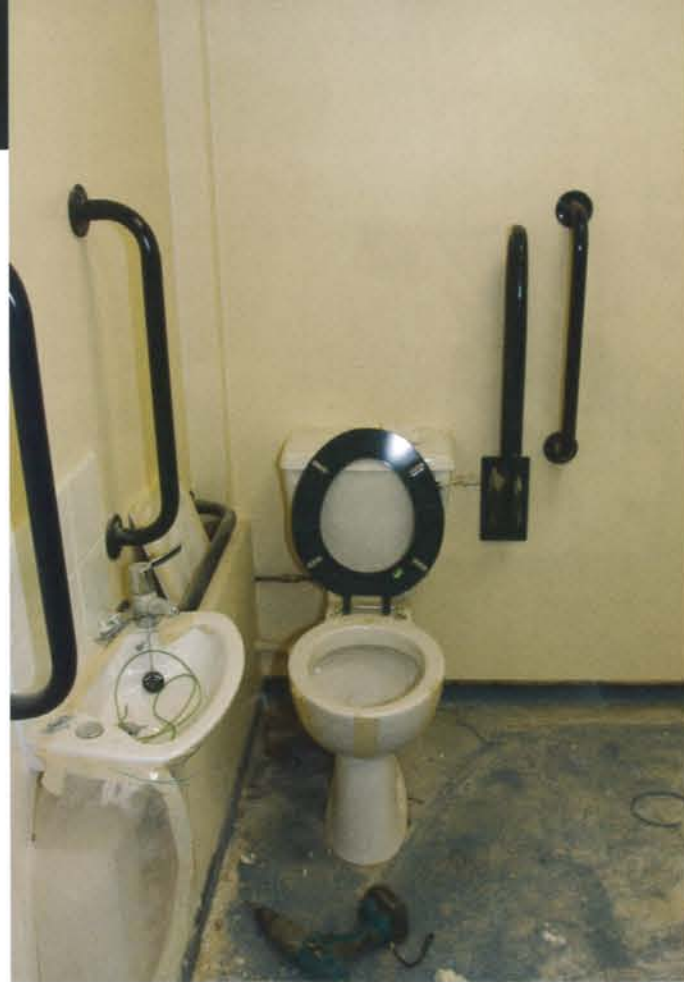
A disabled toilet
