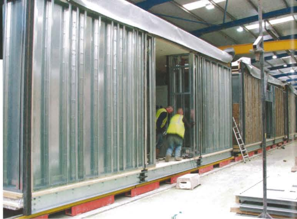
The modular cell units under construction
