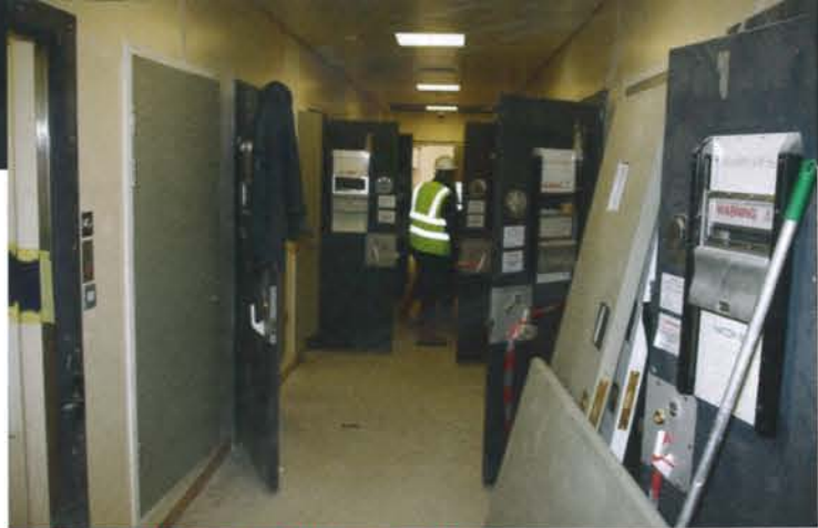
A cell corridor note the Cell Security doors.
