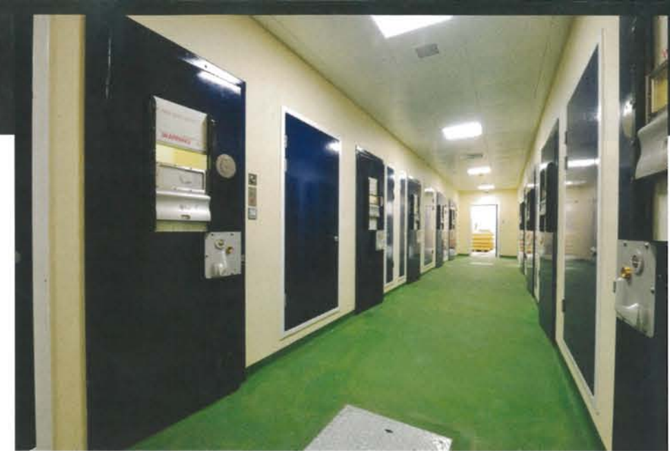
Note the services access door.
