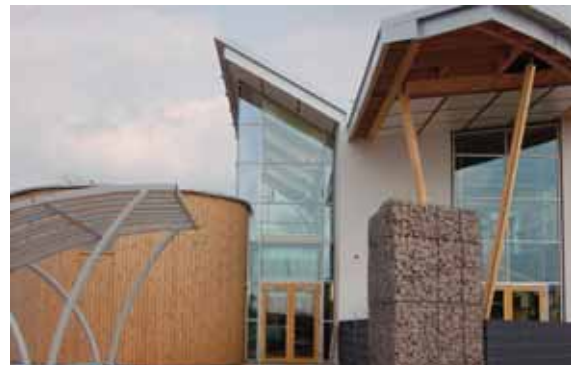
Construction draws to an end on the Wolseley Sustainable Building Centre
